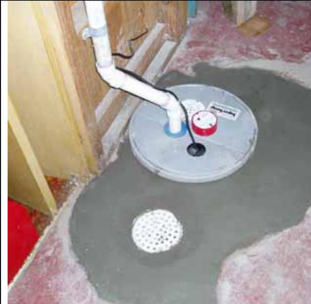
Foundation drains have been disconnected from the sewer and diverted to a sump pit, where it is pumped to the surface. This model has a high water alarm that will alert the homeowner to sump pump failure. If pump should fail, overflow water will run to near by floor drain.
