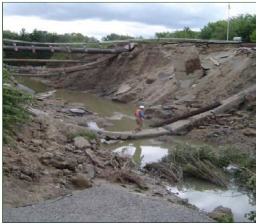
Figure 14: After a Severe Storm Event (August 2005): Eroded Culverts and Road, Finch Avenue: Toronto (D. Haley)
