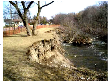
Erosion on Spencer Creek, storm activity, Hamilton, spring 2011
