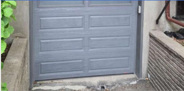
Reverse slope driveway causing a thousand of basement floodings
