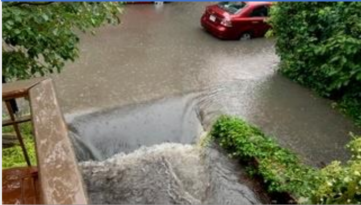
Reverse slope driveway causing a thousand of basement floodings
